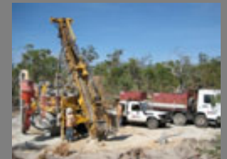
Drilling at Kingsgate
